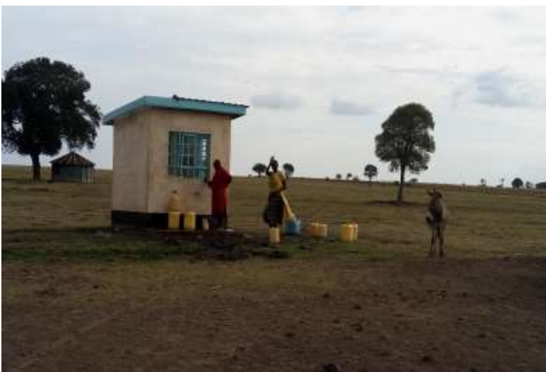
Water At the village center Kiosk
